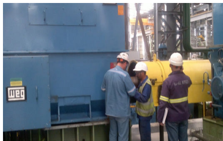
Onsite installation of Earthrings at SAFFEL STEEL
