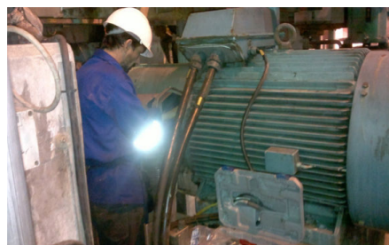
Onsite installation of Earthrings at SAPPI SAICCOR
